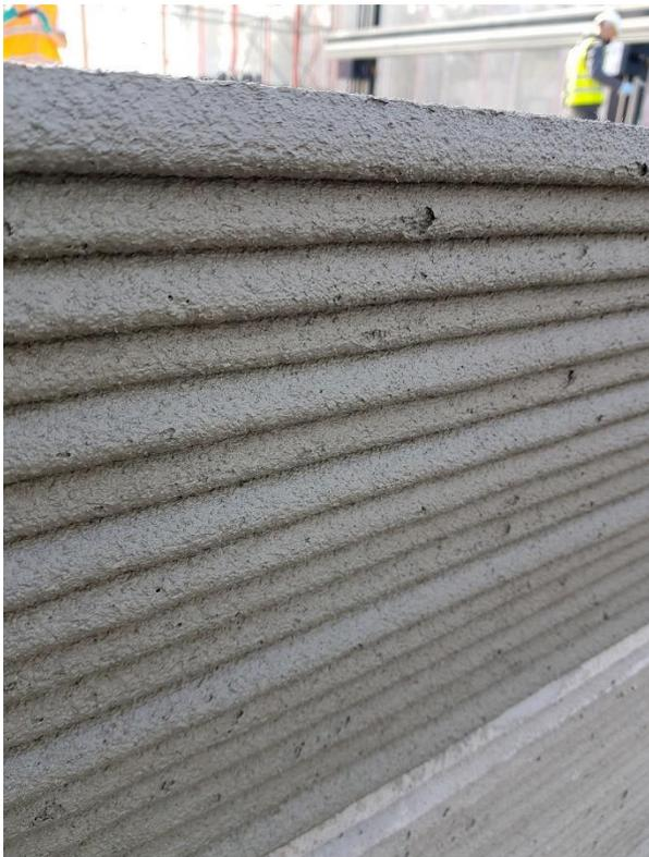
Big challenge. The material for 3D printing had to be easily pumpable and easy to extrude. It must also quickly build up sufficient load-bearing capacity so that the lower layers do not fail under the load of the upper layers. At the same time, it must also ensure the bond between the layers.
